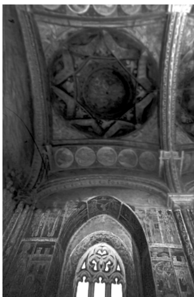
Fig. 6. Similar system of 'stepped arches' supporting a cupola: up, Lviv, Three Hierarchs Chapel, 1591; down, Moldavia, Probota church, narthex, 1530
